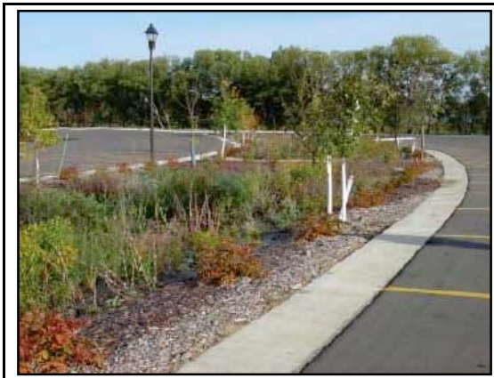
A depressed swale with plants tolerant of wet and dry conditions captures and treats runoff from the adjacent parking areas (examples above and below).
