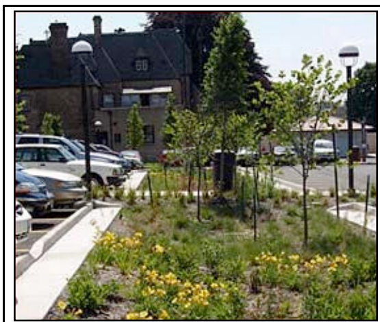
A depressed swale with plants tolerant of wet and dry conditions captures and treats runoff from the adjacent parking areas (examples above and below).
