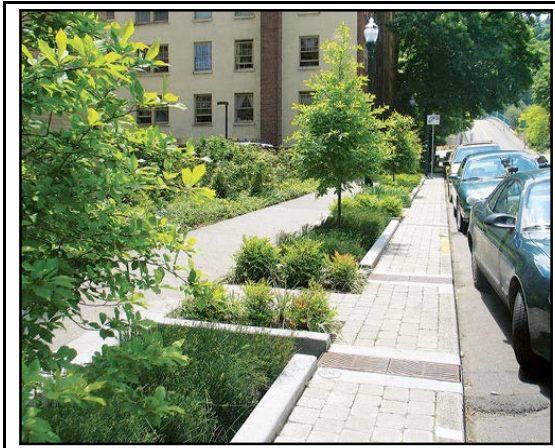
Sidewalk buffer strips intercept runoff before it reaches the street.
