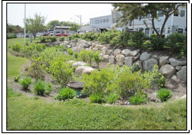
A Bioretention area is a depression with underdrains and plants tolerant of both wet and dry conditions.
