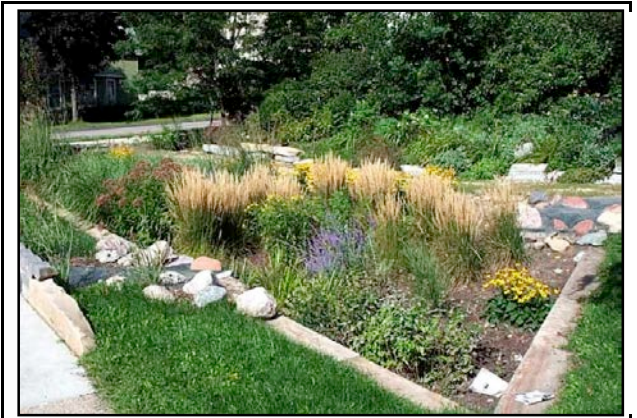
A rain garden is a depression with underdrains and plants tolerant of both wet and dry conditions.
